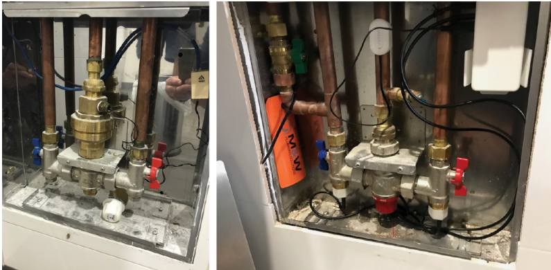
Figure 1: Images depict typical Aquablend TMVs with Smart Flow Monitoring system used within the study.
